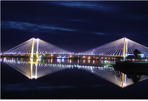
Cable Bridge at night.
